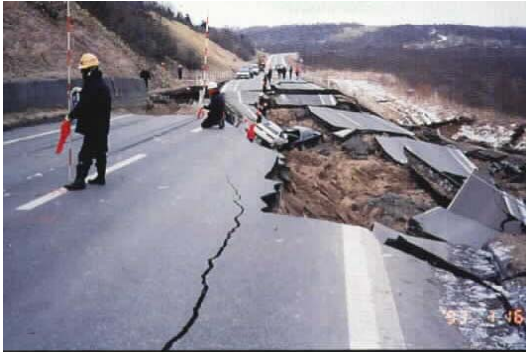
a part of road embankment constructed curved slope was slid away, in 1993 Kushiro-oki Earthquake.
