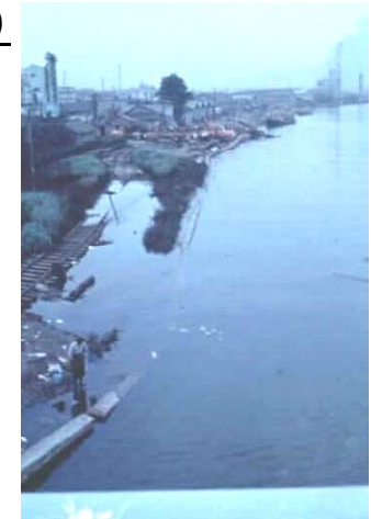
river sides slid toward river with many parallel cracks, in 1964 Niigata Earthquake 河川護岸の側方流動
