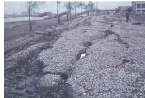
river sides slid toward river with many parallel cracks, in 1964 Niigata Earthquake 河川護岸の側方流動
